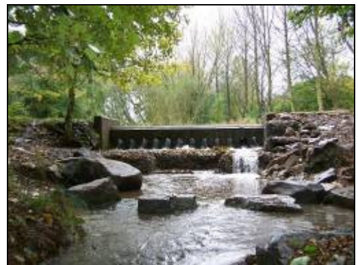
Restored dam by Holly Hayes Pond
