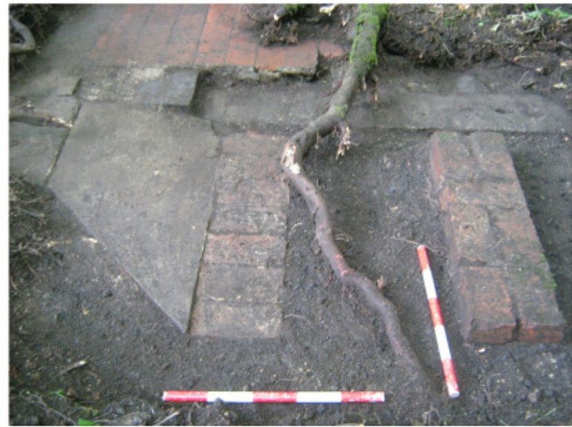
HOLLY HAYES COTTAGES T3 PLINTH AND NORTH WALL JULY 2008
