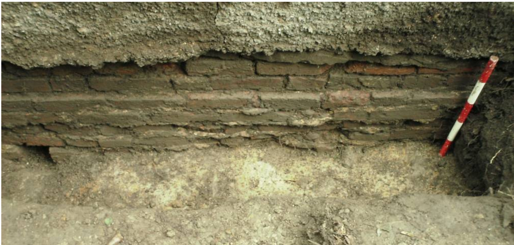
TEST PIT 5 VIEW WEST SHOWING THE FOUNDATION WALL OF HOLLY HAYES FARM HOUSE
